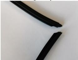
3. Replace the gasket so that "twisted" side looks toward the frame/sash.
